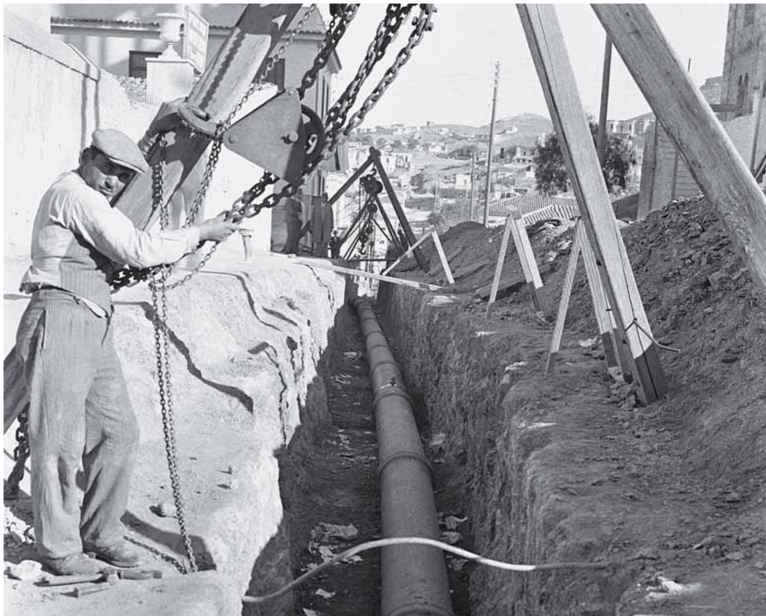
Water supply network construction within the city. 1935
