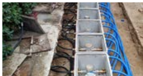
New type water meter shaft system
