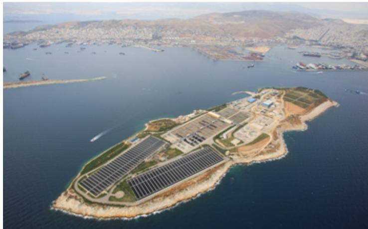
The Psyttalia WWTP is the main wastewater treatment plant in the greater Athens area, receiving an average wastewater flow of approximately 730,000 m<sup>3</sup>/d. The Psyttalia WWTP capacity is 5.600.000 p.e., being one of the biggest WWTPs in Europe and worldwide.
